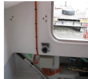
Inside view of water connection
